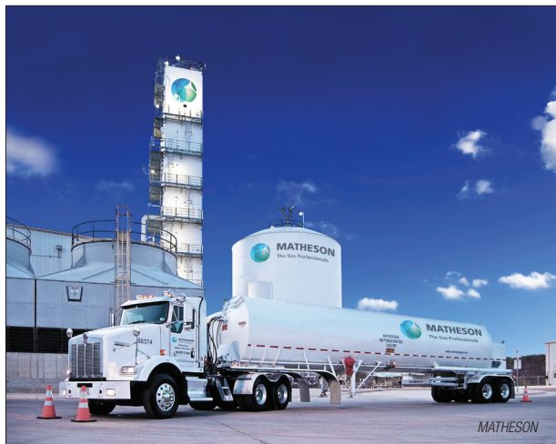
FIGURE 1. Cryogenic distillation in air-separation units, like the one shown here, is a widely used technology to generate large volumes of oxygen and nitrogen
